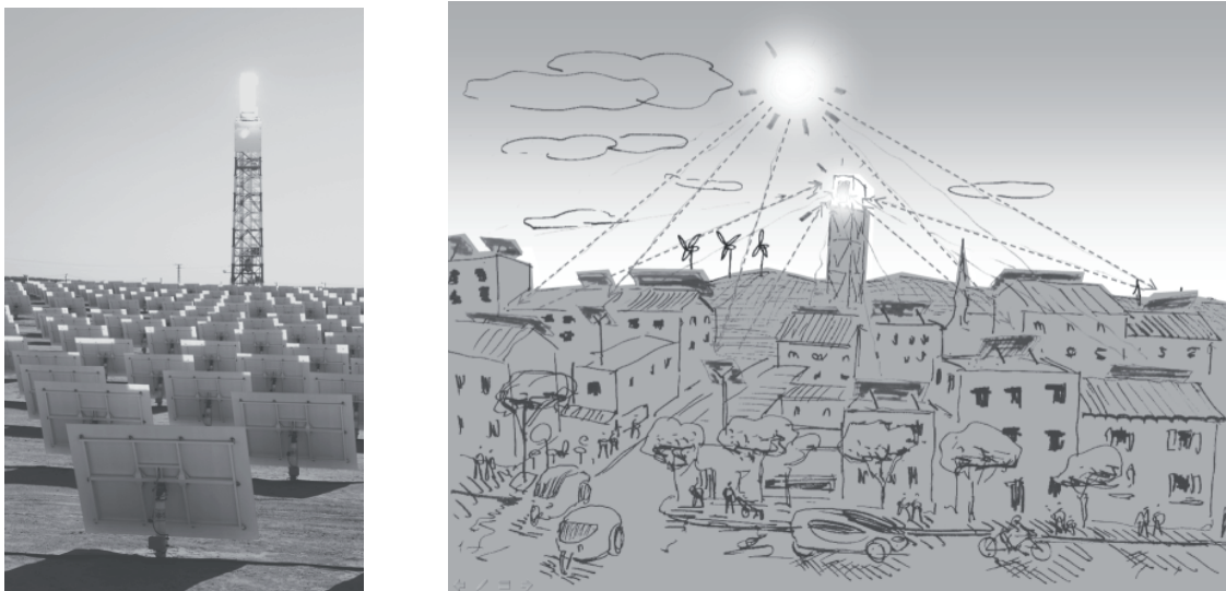
On left, photo of a solar thermal plant in the desert of Mojave: mirrors focus solar rays on the tower and produce heat at high temperature and then electricity with a steam turbine (BrightSource Energy) On the right (Menard, 2010), heliostats (mirrors which turn so as to keep reflecting sunlight toward a target) are installed on existing roofs and focus to the tower: the hub for the heating district network and electrical plant.
