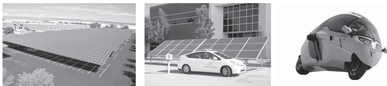
Left, the Bell PV-car park in Albuquerque (New Mexico, USA): 1,600,000kWh of electricity a year on 2 hectares of parking area. In the middle, a plug-in hybrid, the Prius 3, connected to PV-panels for reload. Right, a 2“wheel car”, X-Prize winner 2008 during the Zero Race in 2010: the shape as a lever for efficiency.
